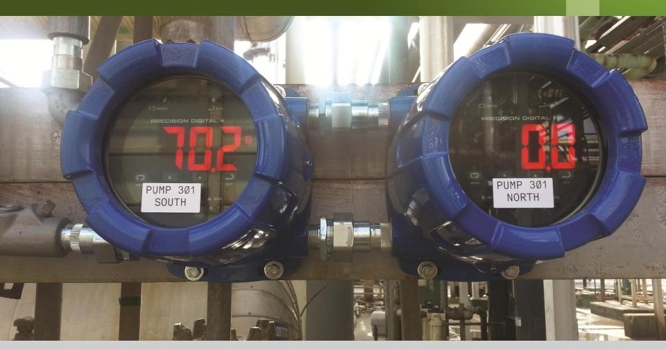
Explosion-proof pump controllers with huge displays and built-in pump alternation control.
